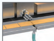
Removal of large amount of dust created through dividing boards
